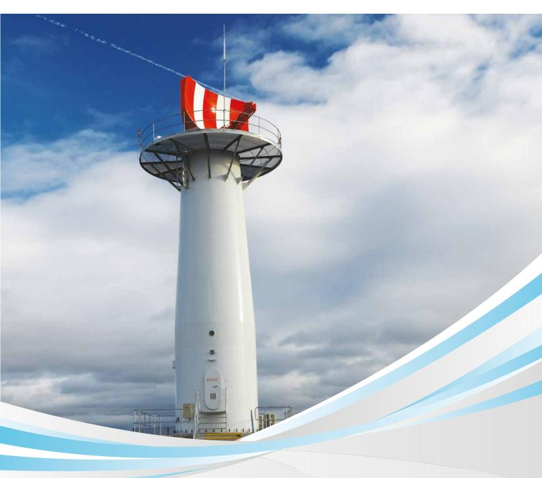
Advanced S-Band Solid-State Primary Surveillance Radar
